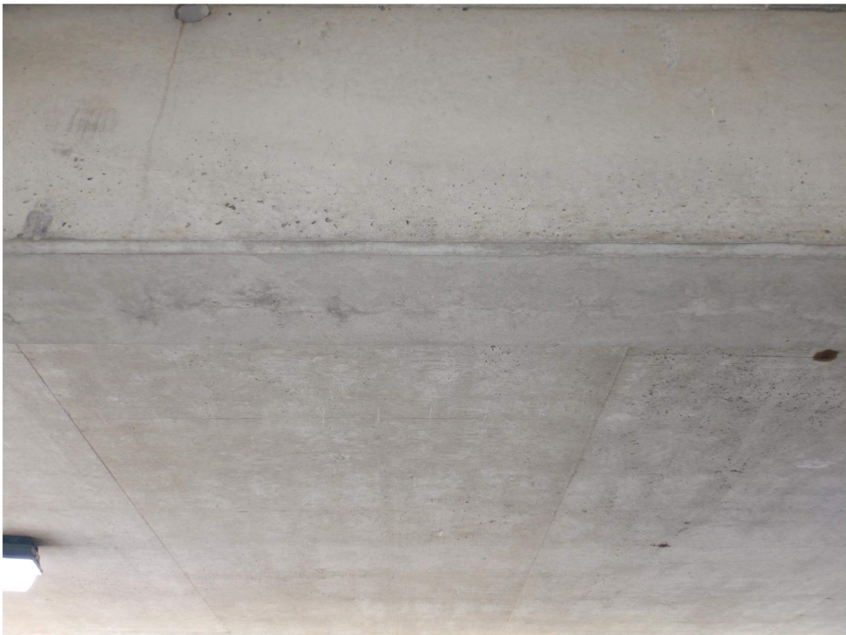
level6-ei-underside of beam
