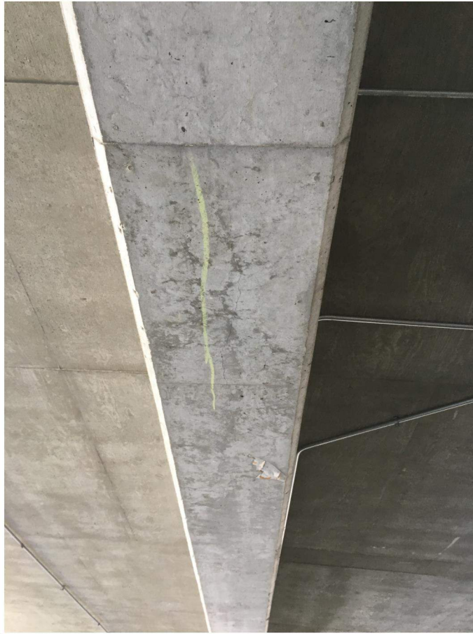
level3-ei-underside of beam
